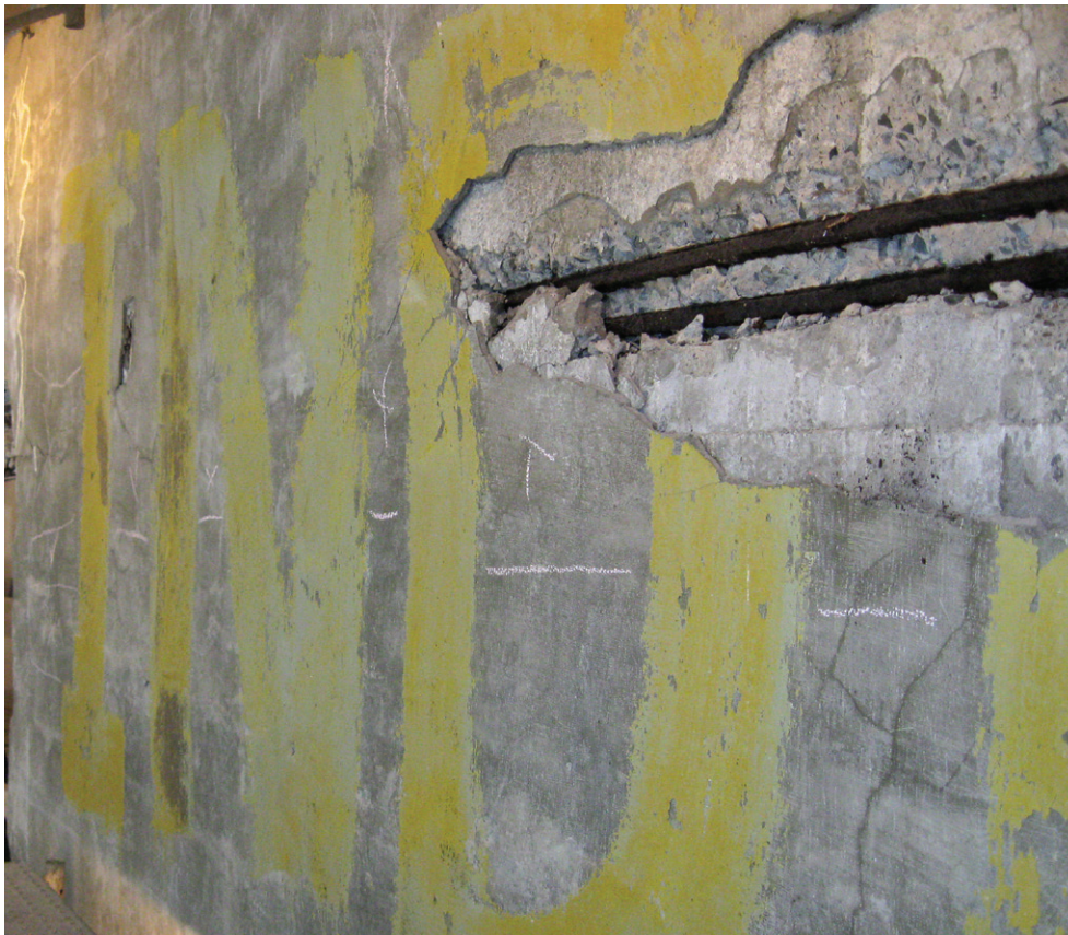
Typical conditions at locations of Political Statement prior to concrete repairs, 2014.
