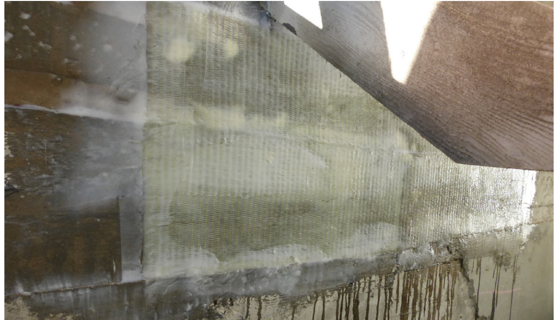
Quartermaster Building conditions during construction including (top) the cold joint revealed during parge coat demolition, which was repaired through the exterior application of FRP (below), which was then concealed behind the new parge coat.
